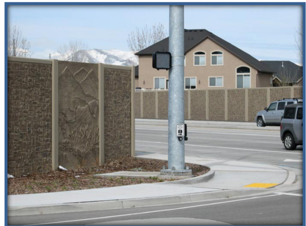
PIONEER CROSSING BLVD SOUND WALL, LEHI
