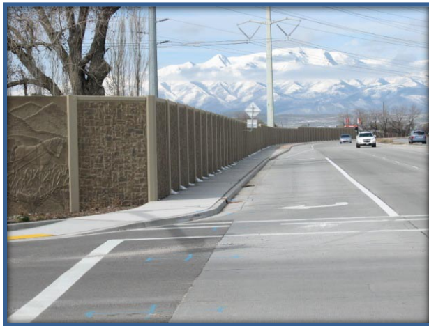
PIONEER CROSSING BLVD SOUND WALL, LEHI
