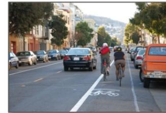
A bike lane is a portion of the roadway that has been designated specifically for bicycles by striping, signage, and pavement markings. Bike lanes enable bicyclists to ride at their preferred speed without interference from prevailing traffic conditions and facilitate predictable behavior and movements between bicyclists and motorists (NACTO). Bicycle lanes are typically best used on major roads, provide direct access to key areas, and include one-way travel.
