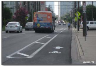
Buffered bike lanes are conventional bicycle lanes paired with a designated buffer space separating the bicycle lane from the adjacent motor vehicle travel lane and/or parking lane (NACTO).
